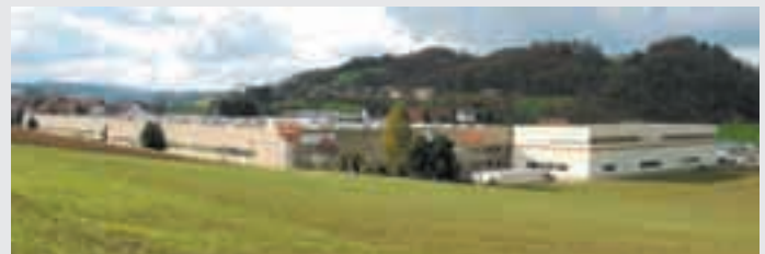
Busch Manufacturing Plant – Switzerland
